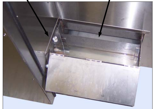
Reservoir Tank Cabinet (lid open)
